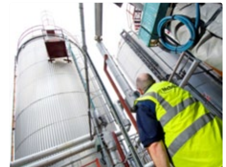
Middleton raw material storage vessel
